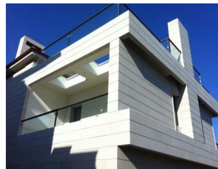
Figure 5. External wall with cut stone.
